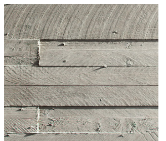
6. BOARD FORMED CONCRETE
