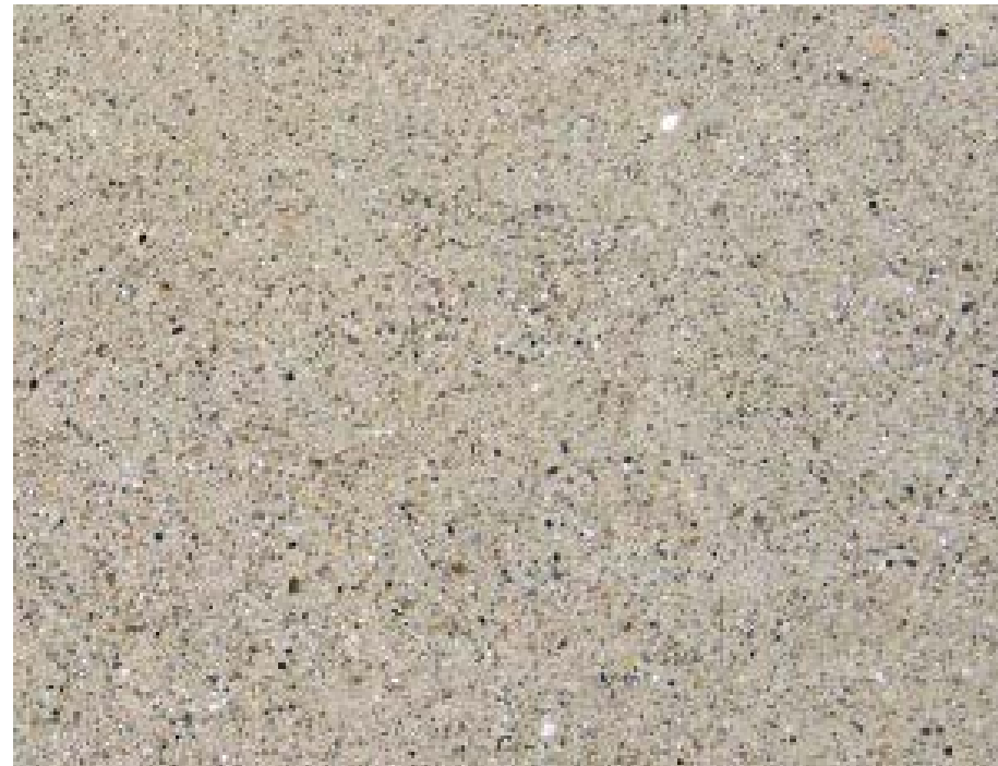
PAVING INTEGRAL COLORED CONCRETE
